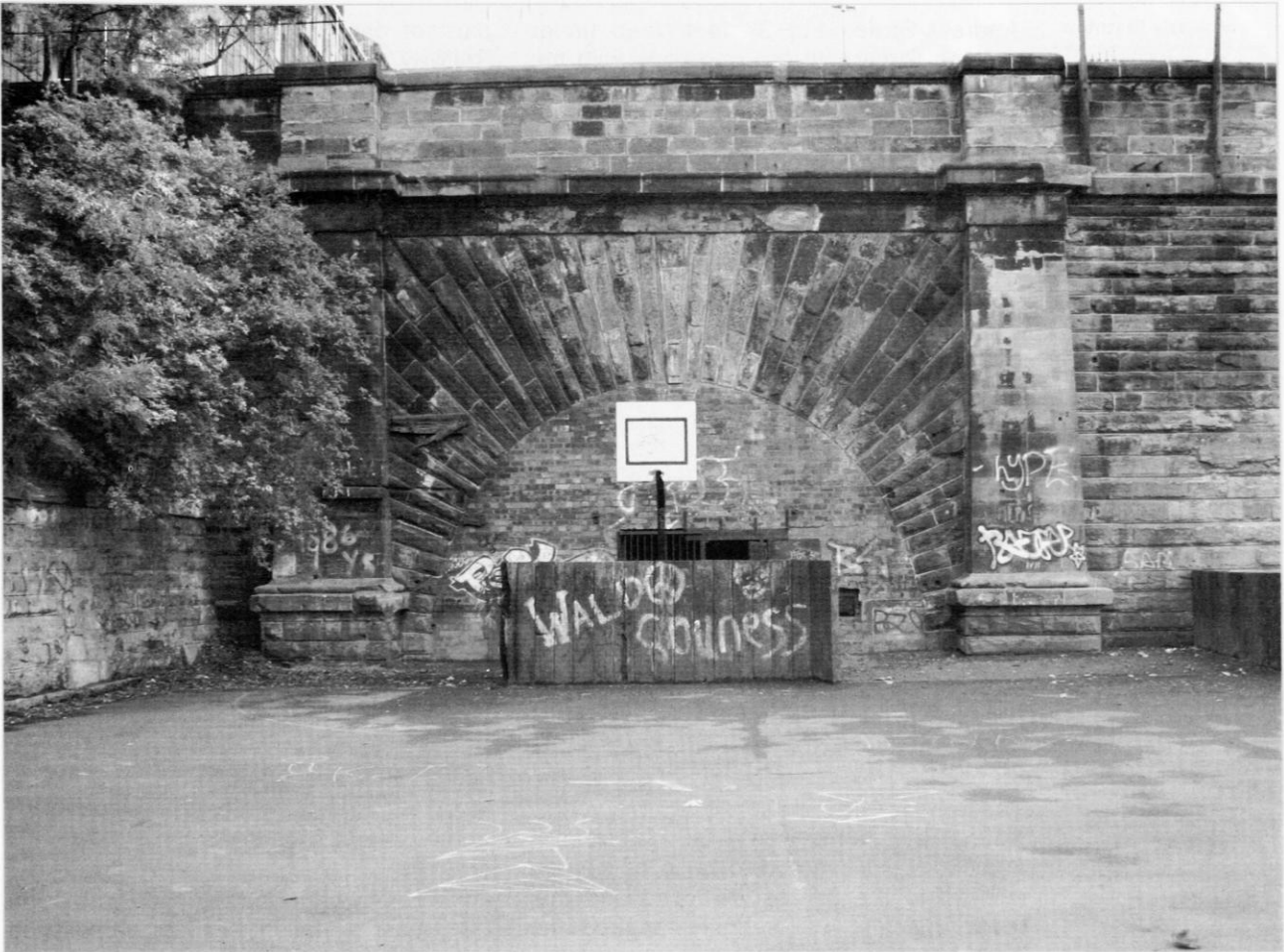
The North portal of Scotland Street tunnel - photo by Nick Catford
